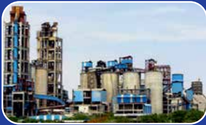
CEMENT PLANT MUKTYALA
